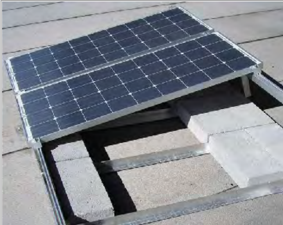
Figures 5 - 8. Examples of Ballasted PV Racking
