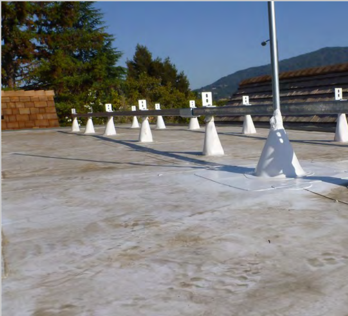
Figures 2. and 3. Examples of TPO Booted PV Mounts.
