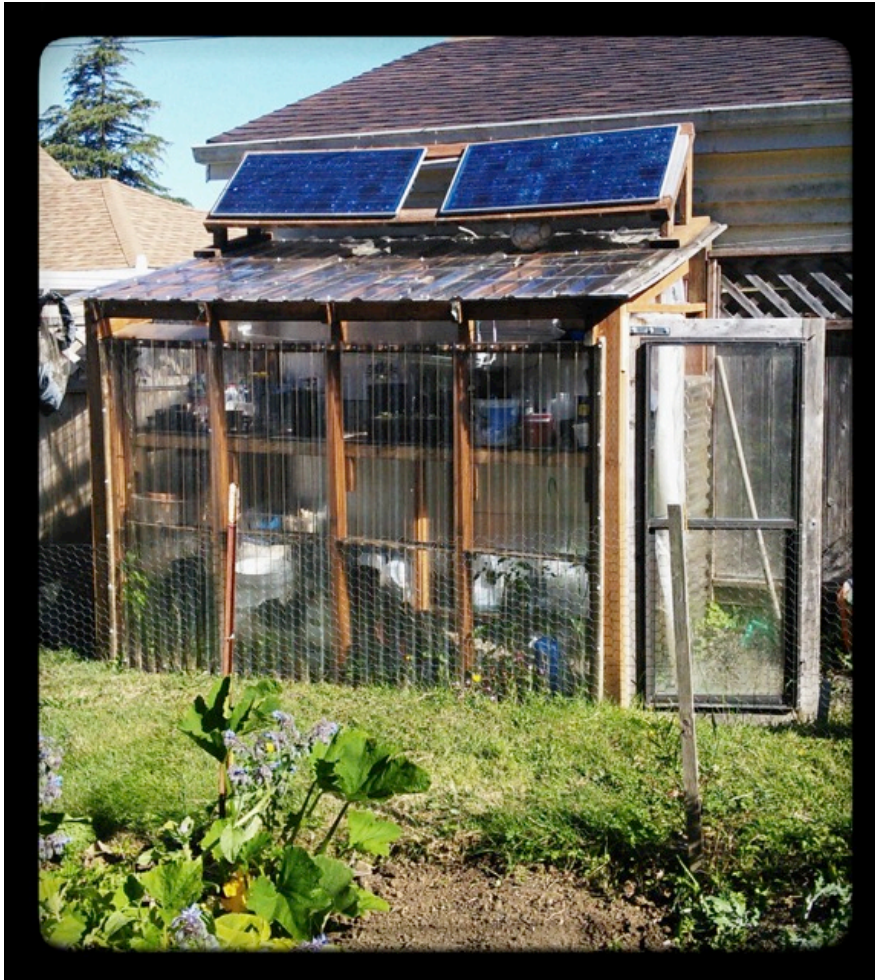
Solar Powered Greenhouse with 2 refurbished 64-Watt Photovoltaic modules. See “Off-Grid Systems Handout” for photos of the two off-grid systems.
